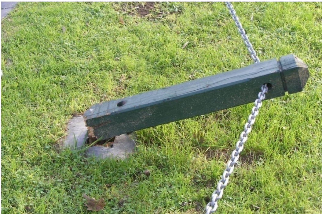
Figure 33: A fused post which has obviously broken at the base instead of at the fused location identified by the drilled hole.
